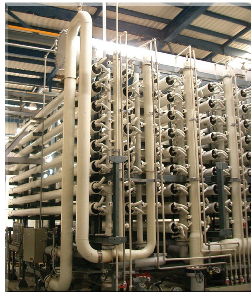
SWC3 membrane installation, 45 MGD (170,000 m³/d) in Fujairah, U.A.E.
